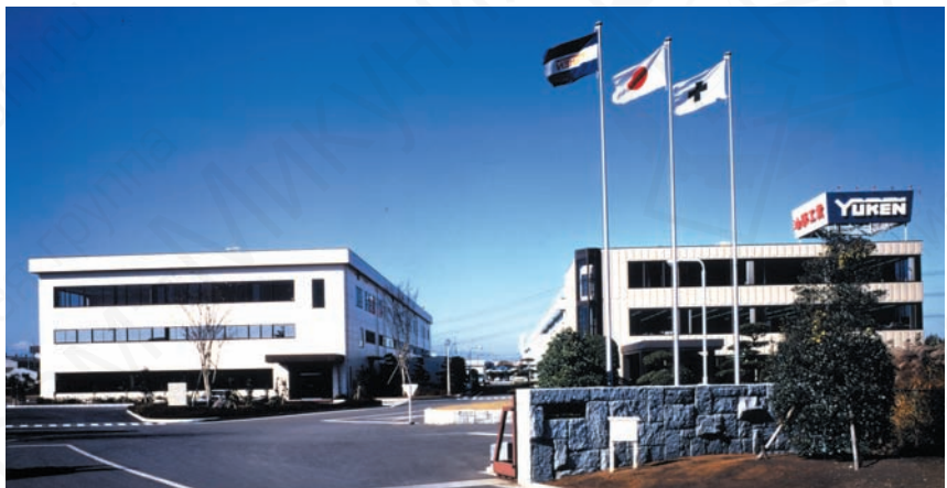
● Sagami Plant Front Gate
